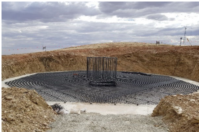
Figure ES.8 Wind turbine foundation
