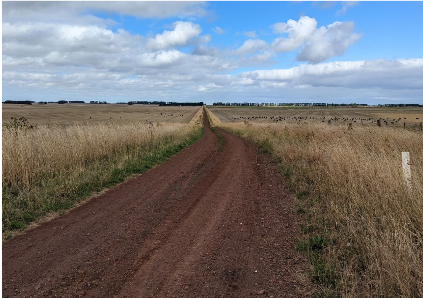
Western end of Immigrants Lane, near intersection with Woolsthorpe-Hexham Road. Existing gravel roads in the area appear to be generally constructed with basalt or scoria gravel.
