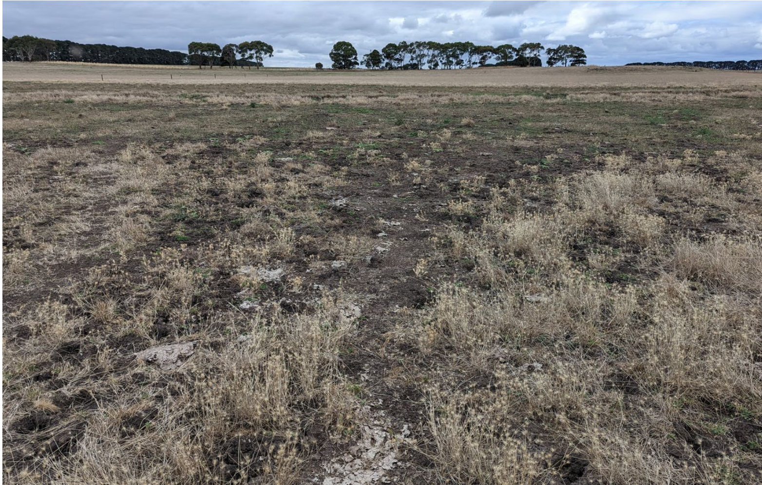
Swamp soil deposit adjacent to proposed WTG T153. Underground cable and site access road proposed to cross the deposit. Soil is dark grey high plasticity clay with high dry stiffness, but inferred to lose stiffness rapidly with saturation.
