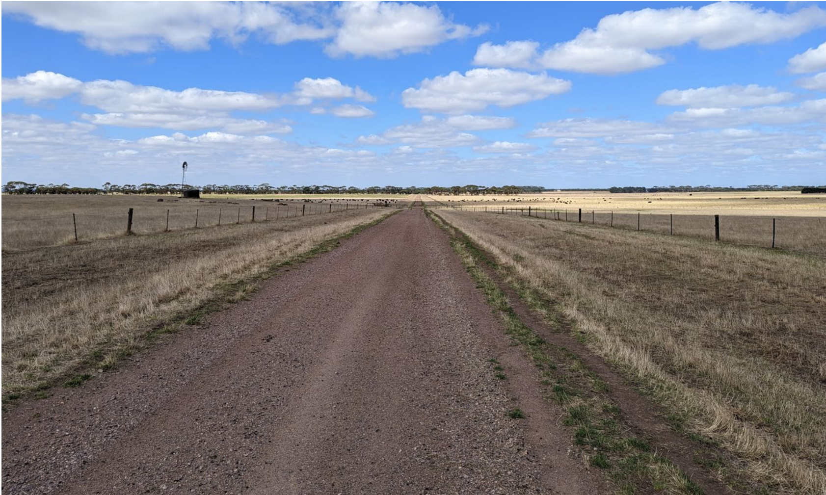
An internal farm road close to proposed WTG T20. Gravel roads in the area were generally in good condition, noting that the site visit was undertaken in early March after a relatively dry January and February.
