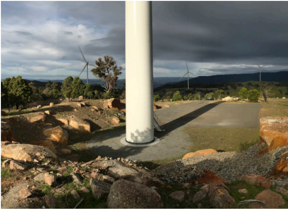
Image 3 Crane Hardstand Area (Source: NGH)
