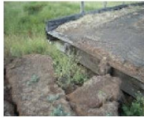
BURCHETT CREEK BRIDGE SOHE 2008
