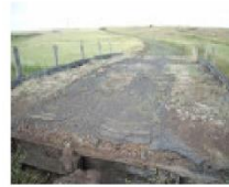
BURCHETT CREEK BRIDGE SOHE 2008
