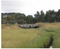
BURCHETT CREEK BRIDGE SOHE 2008
