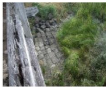
BURCHETT CREEK BRIDGE SOHE 2008
