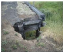
BURCHETT CREEK BRIDGE SOHE 2008
