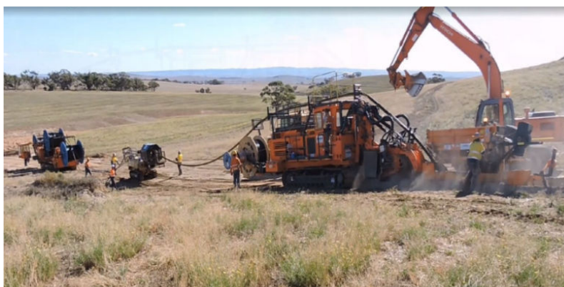
Figure 6.24 Example of wind farm cable trench laying (Source: TESMEC, 2019)
