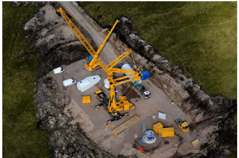
Figure 6.4 Aerial view of typical wind turbine hardstand during construction (Source: Wind Prospect)
