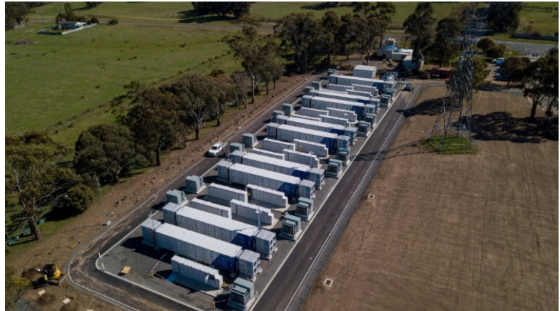
Figure 6.10 Example 30-megawatt battery energy storage system at Ballarat, Victoria (Source: DEECA, 2025c)
