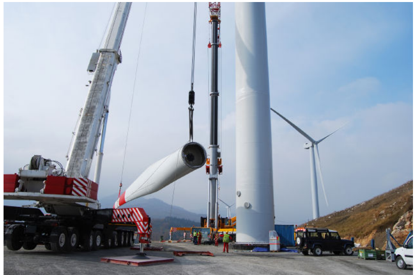
Figure 6.6 A blade being lifted onto a wind turbine
